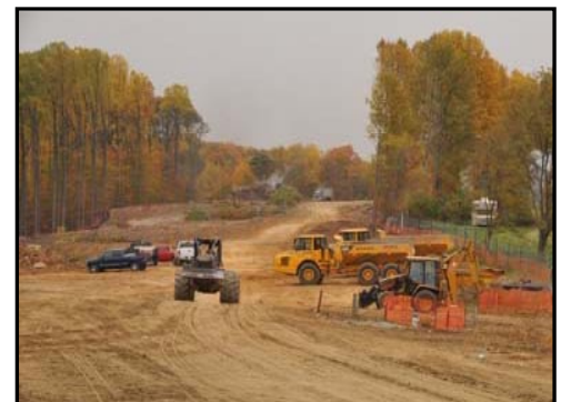
Clearing the right-of-way east of US 29 in Contract C.
