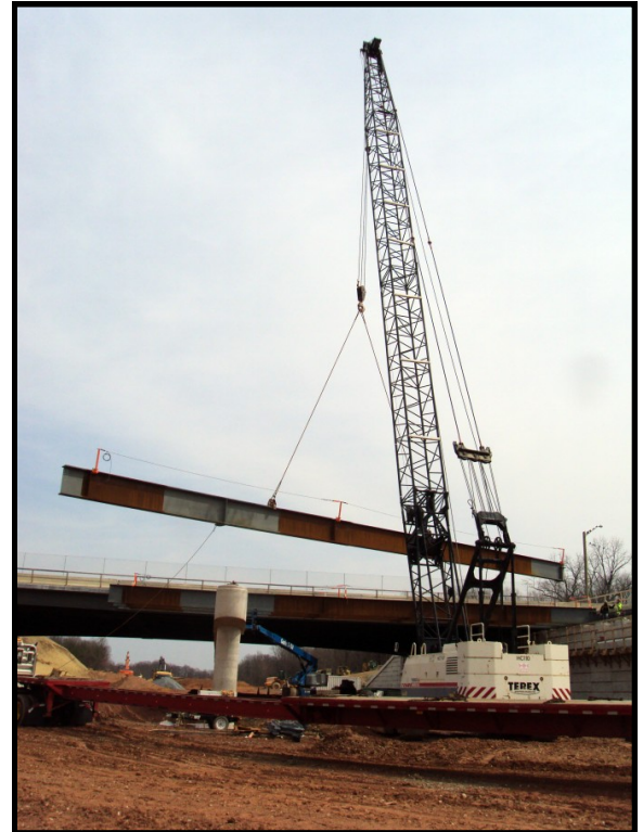
Setting steel girders for New Hampshire Avenue Bridge
