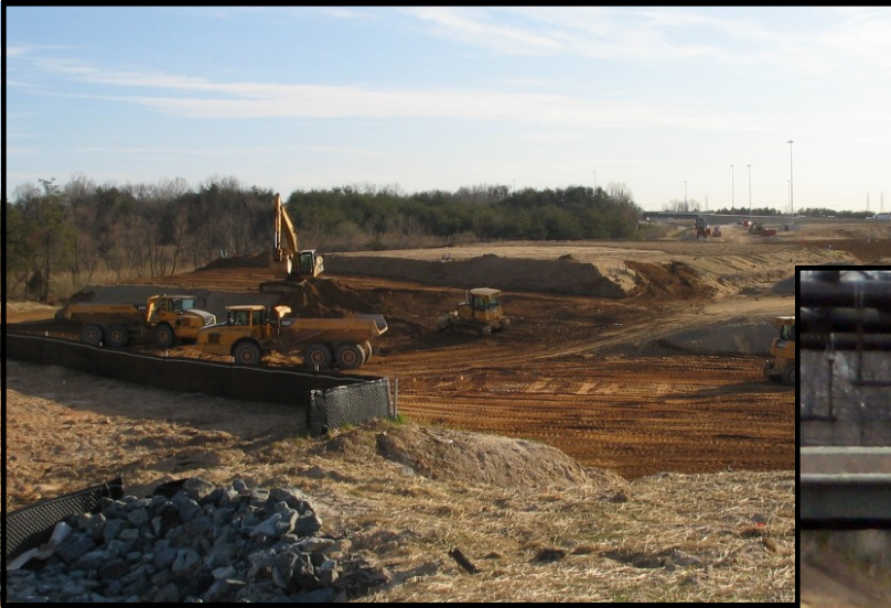
Grading west of I-95 Interchange
