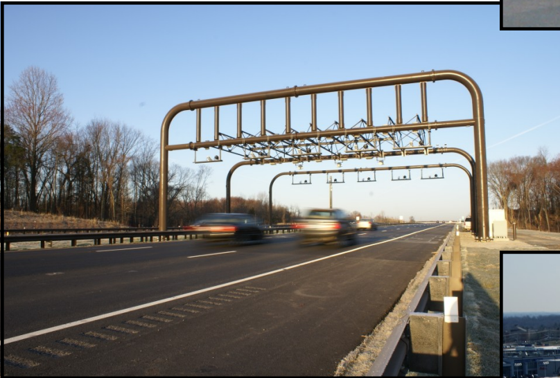
Traffic going through the toll gantry
