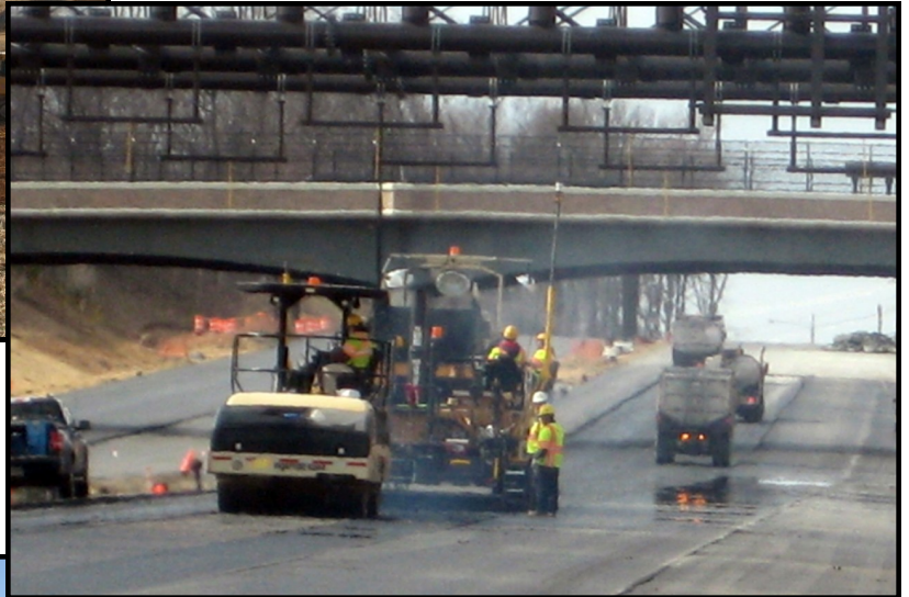
Placing hot-mix asphalt (HMA) for mainline pavement
