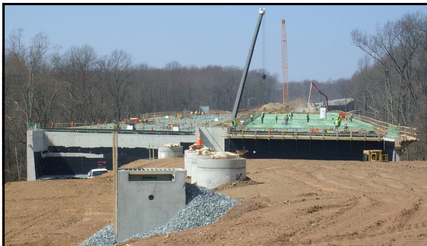
Gum Springs—Paint Branch Bridge
