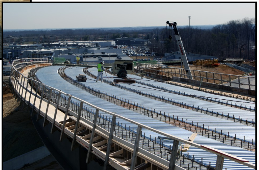
Deck form installation at US 29 interchange
