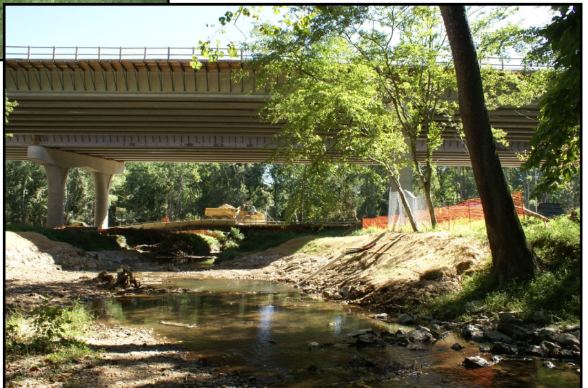
Right: NW Branch Stream Restoration under BR 29
