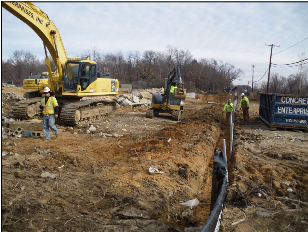
Demolition along US 1 for Eastern Operations Facility
