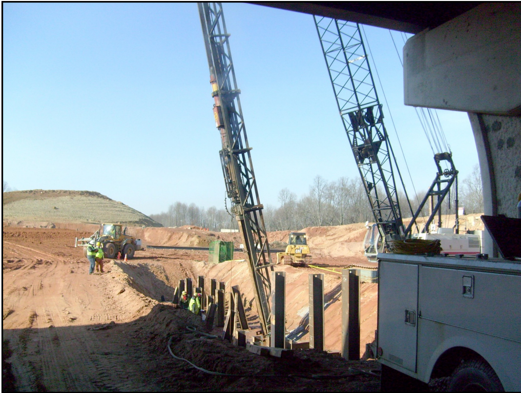
Pile driving At New Hampshire Avenue Bridge.
