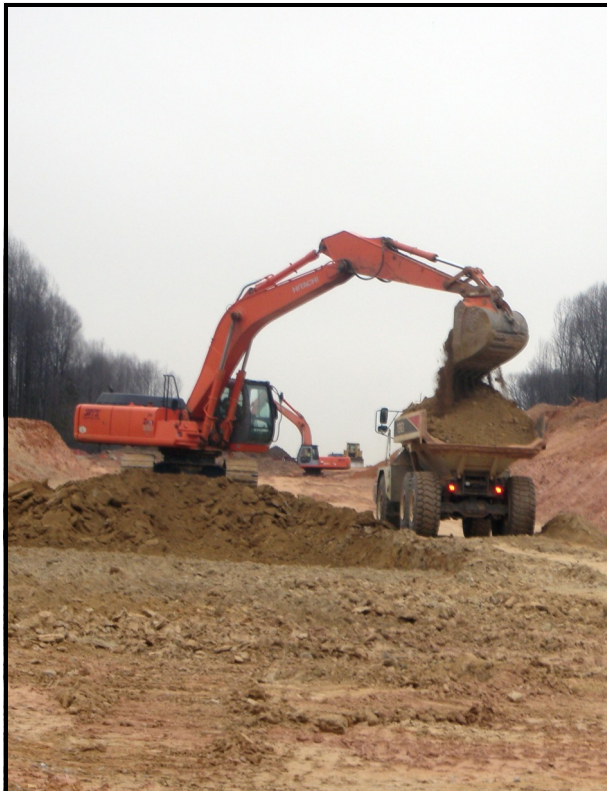
Excavation east of Notley Road
