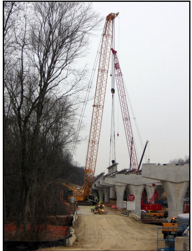
Setting girders for Gum Springs-Paint Branch Bridge
