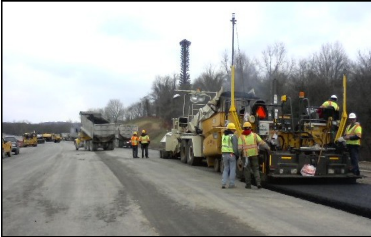
Grading the ICC mainline at Longmead Crossing Drive Bridge
