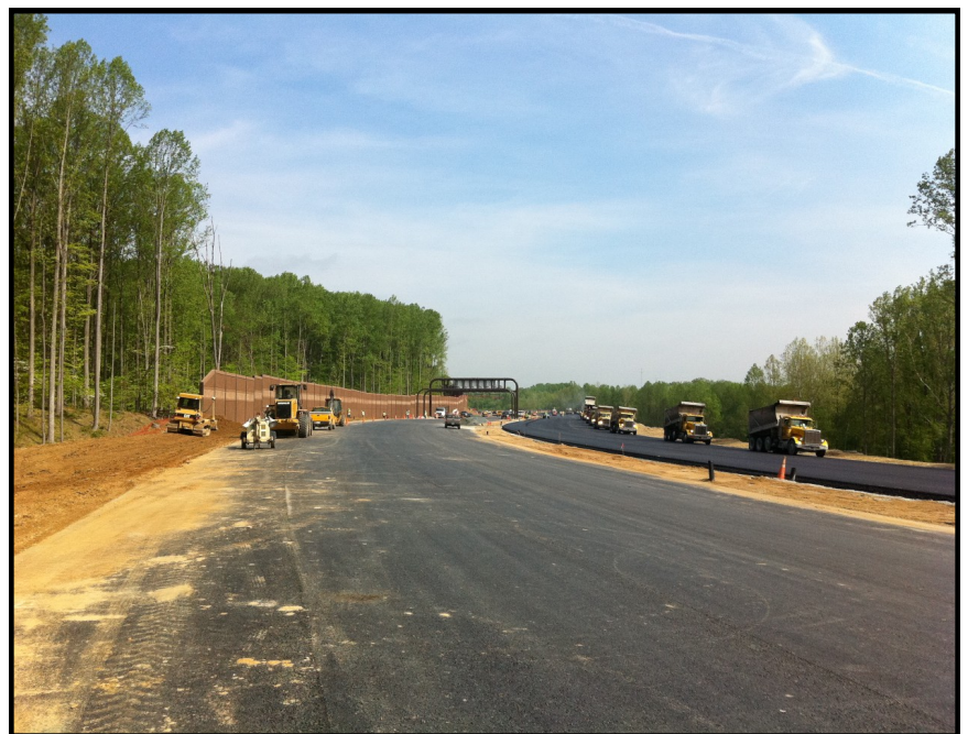
Paving east of Bonifant Road
