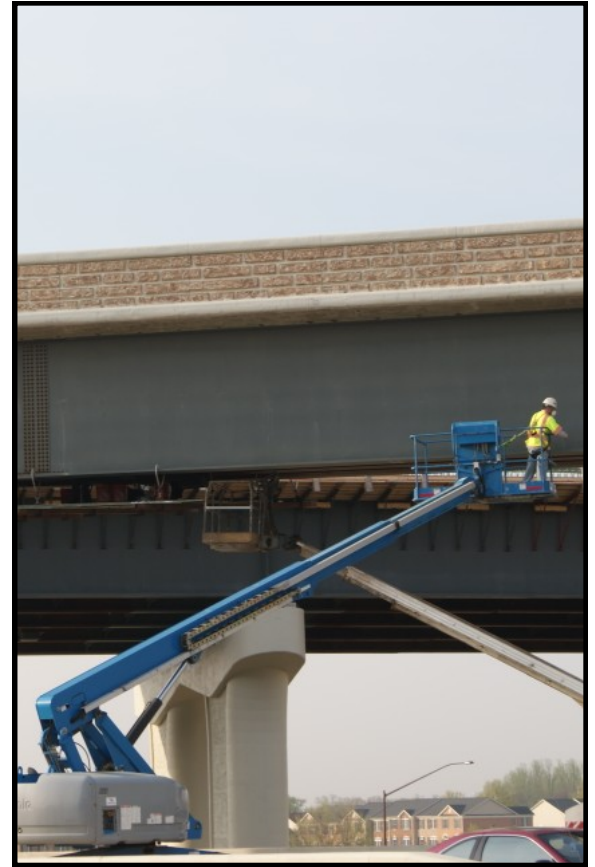
Prepping bridge at US 29 for painting
