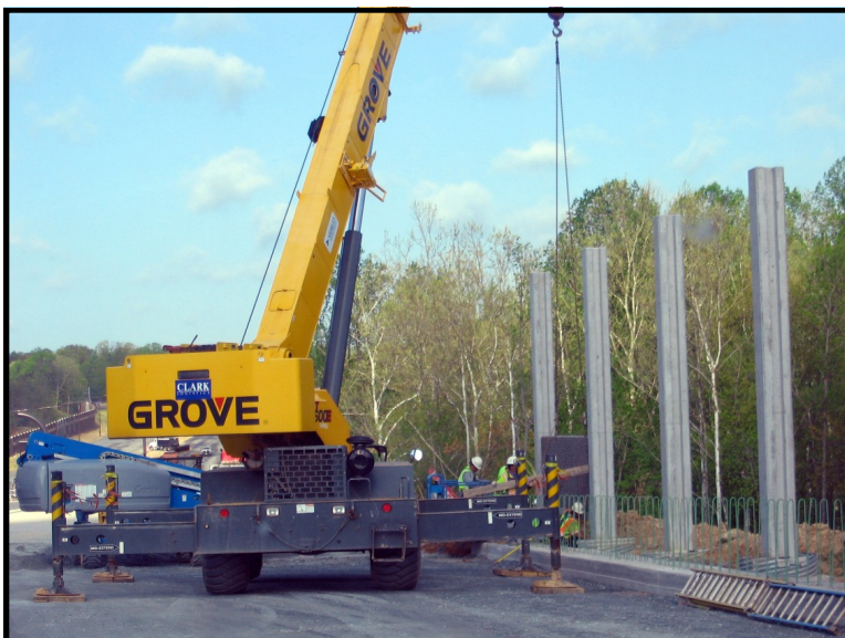
Installing sound barrier panels west of Old Gunpowder Road
