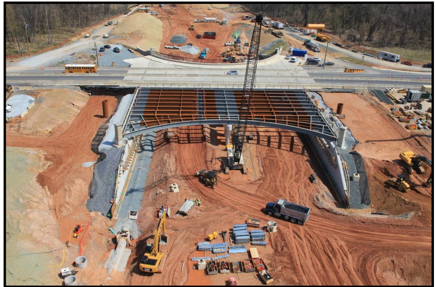
Phase 2 of the New Hampshire Avenue Bridge
