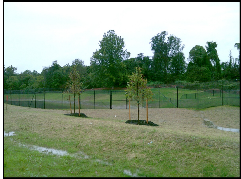
Stormwater management pond west of Bonifant Road
