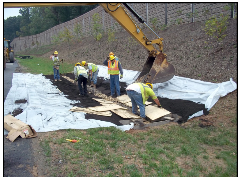
Linear sand filter construction
