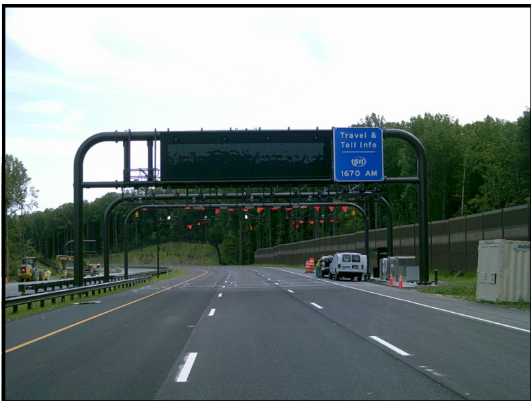
Toll gantry east of Bonifant Road
