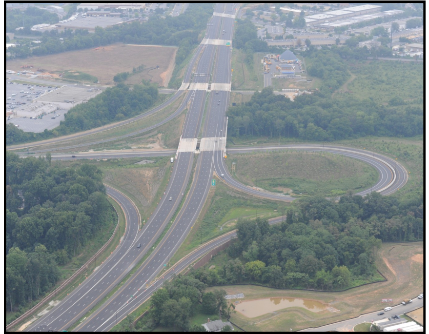
Aerial shot of Contract A
