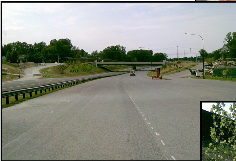
Layhill Road Bridge over the ICC mainline
