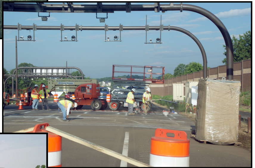
Installing gantry loops west of Old Gunpowder Road
