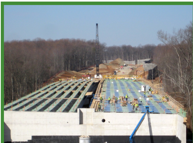
Bridge over Gum Springs-Paint Branch
