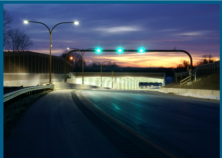
The view looking east towards Georgia Ave on Day One
