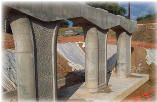
Redland Road Bridge Construction
