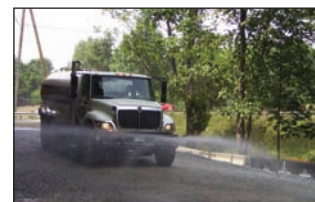
Water truck helping to control dust.
