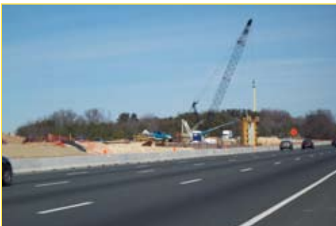
I-95 median bridgework looking North
