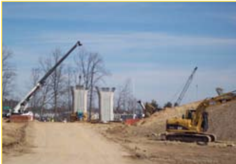
Bridgework on US 29
