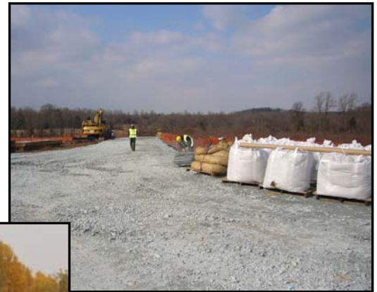
Contract C: (Left) clearing the right-of-way east of US 29.
