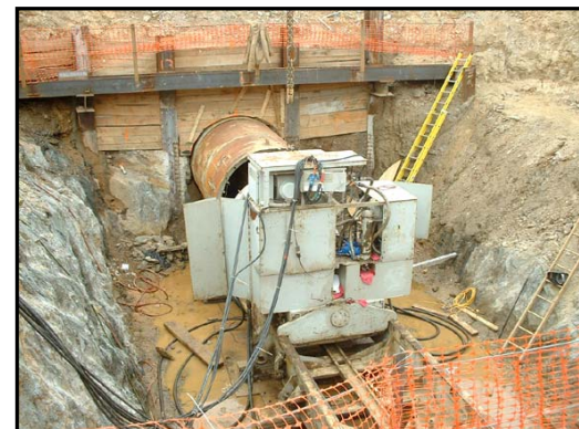
Photo 3- Contract C: 72-inch storm drain is installed under US 29.
