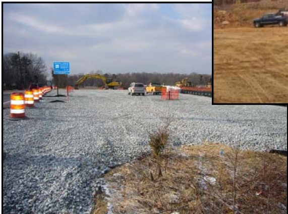
Contract B: (Above) Staging area west of Norbeck Rd.
