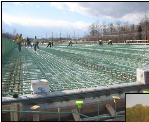
Contract A: (Above) Rebar installation at MD 97 (Georgia Ave.) northbound bridge.
