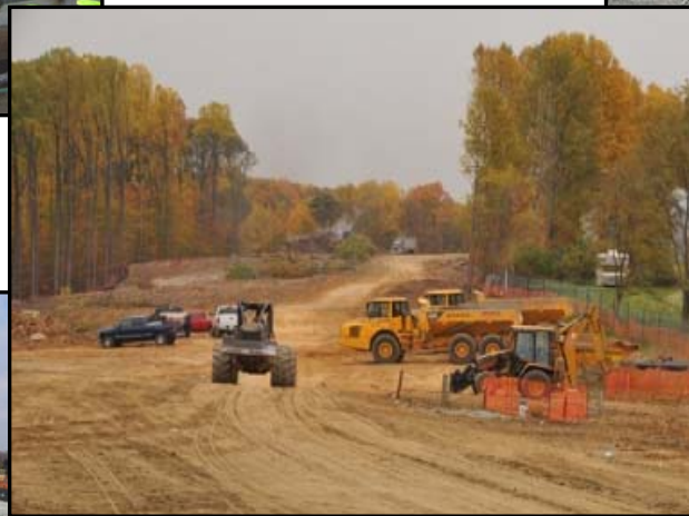
Contract B: (Right) Access road heading west from Norbeck Rd. en route to a stream diversion for a Northwest Branch tributary. Sand bags stand ready (right) for deployment.
