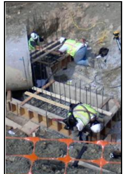
Forming footer at headwall for 60-inch pipe in Contract C.
