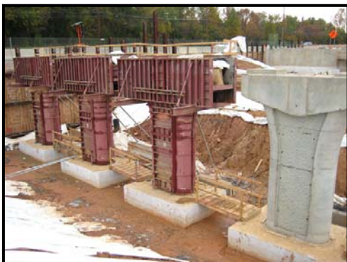
Pier formwork on MD 97 Bridge in Contract A.
