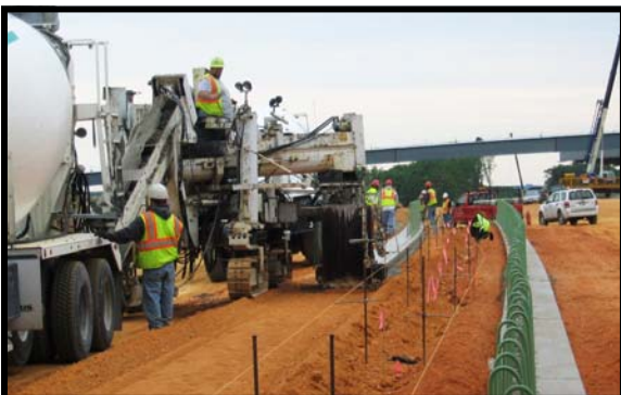
Slipform machine in use near I-95 Contract C
