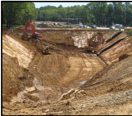
Excavation for 42" waterline west of Norbeck Road Contract B
