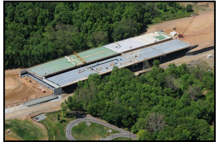
South view of Northwest Branch Bridge Contract B
