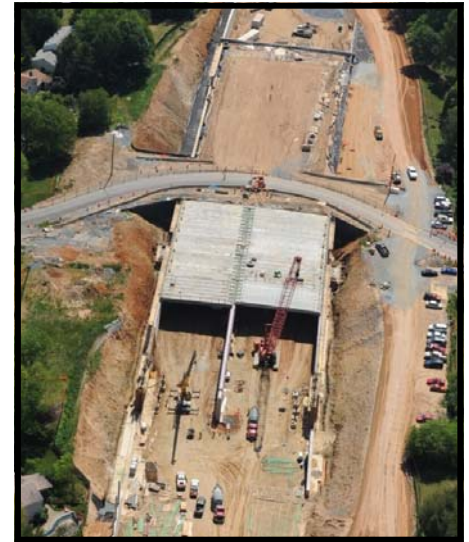
East portal of Olde Mill Run deckover
