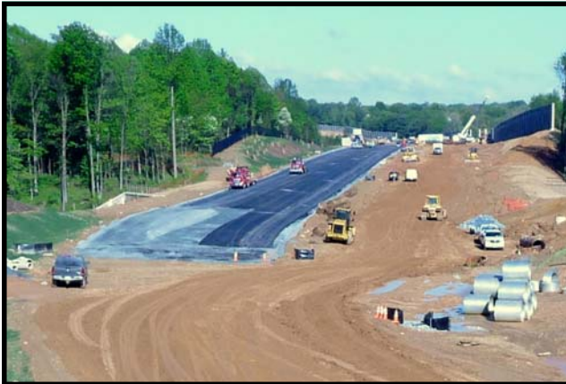
ICC Mainline paving west of Redland Road Contract A
